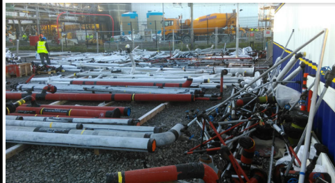
Congested pipe laydown area
