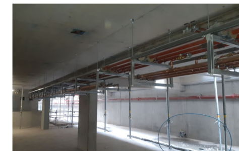
Mock up piperack modules in basement
