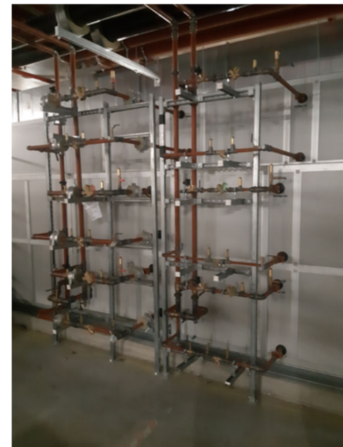
Valve sets installed on site connected to Air handling units
