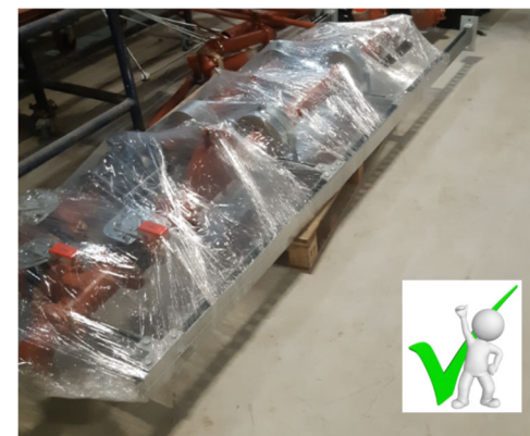
Prefabbed valve set delivered to site c/w Unistrut supports
