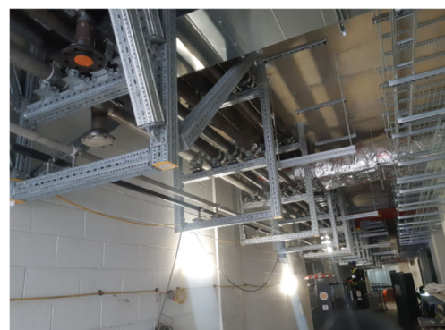
Diagonal bracing at anchor point for Steam
