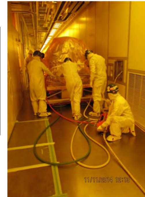
Sensitive equipment being moved using air skates
