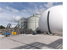
Anaerobic Digestion (AD) Facility consisting of Screening, Grit Removal and Cooling systems. 2no. Buffer Tanks (circa 1000m<sup>3</sup> each), 4no. Primary Anaerobic
