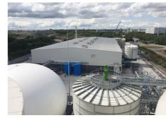
Waste Water Treatment Plant -Treatment of redundant substrate, dewatering, aeration, scrubbing so that the substrate can be introduced back into the foul waste stream . (image on front page).
