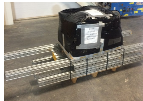
Each delivery has ID label linked to specific site location
